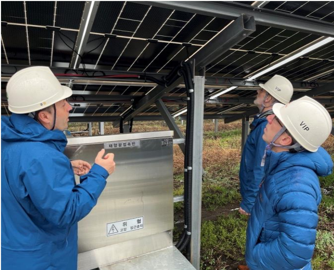
Glennmont on site with correct PPE
