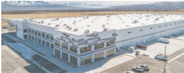
Mountainview Industrial, Salt Lake City, UT Acquired: March 2025
