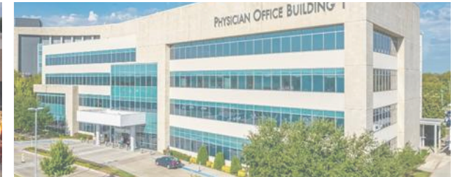
McKinney Medical Office Building, Dallas, TX Acquired: August 2022
