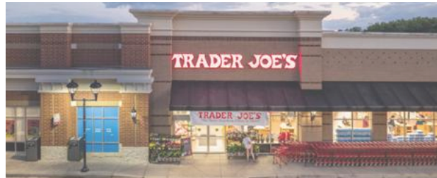
Short Pump Station, Richmond, VA Acquired: December 2024
