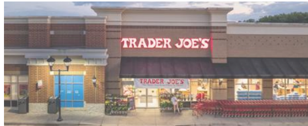
Short Pump Station, Richmond, VA Acquired: December 2024
